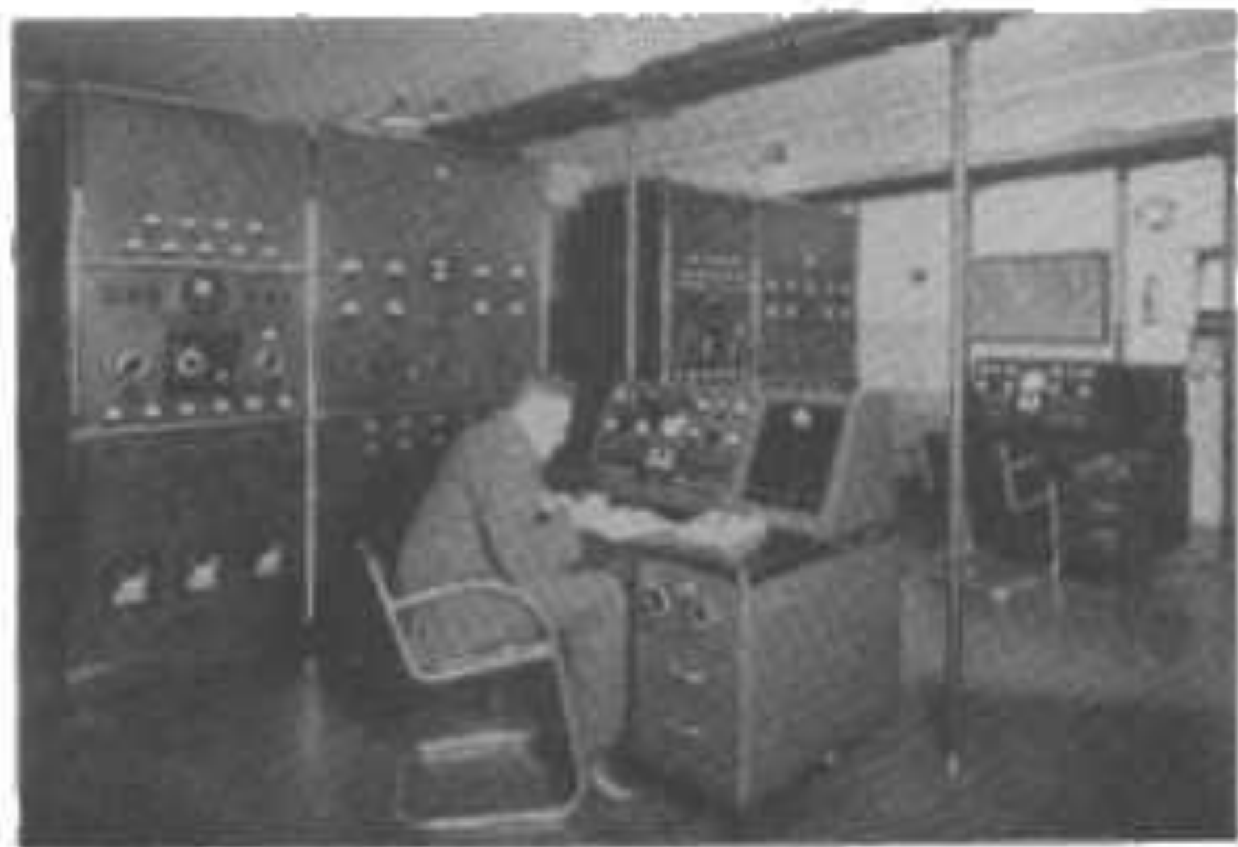
Fig. 9. East Coast CH transmitter room
