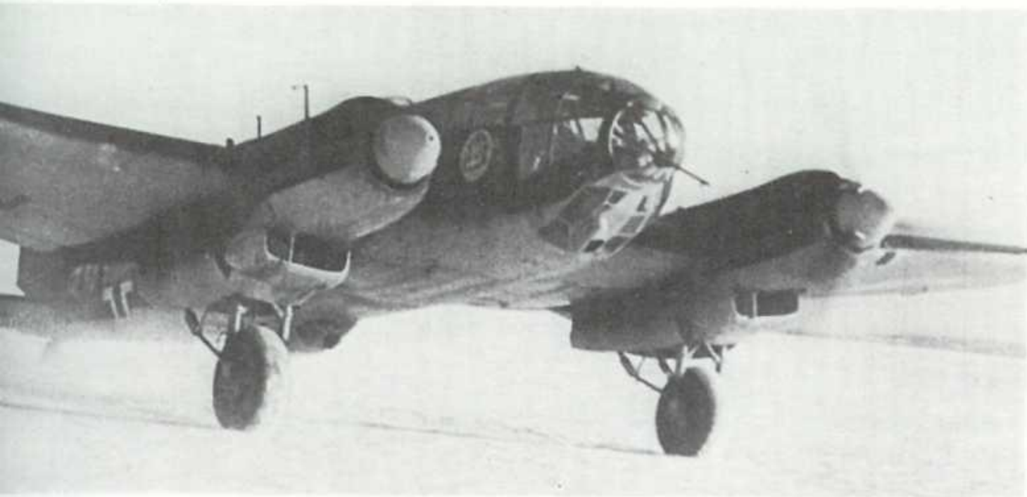
A Heinkel 111 KGr100, probably photographed in Norway where the unit was stationed before their attacks on England. The Viking ship emblem of KGr100 can be seen on the side of the cockpit. The aircraft is equipped with X-Geräte and the additional aerial mast is clearly visible.
